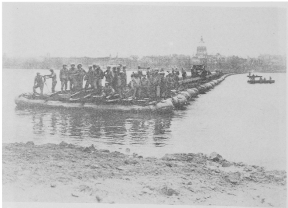
Final construction on the Rhine river at Mainz
