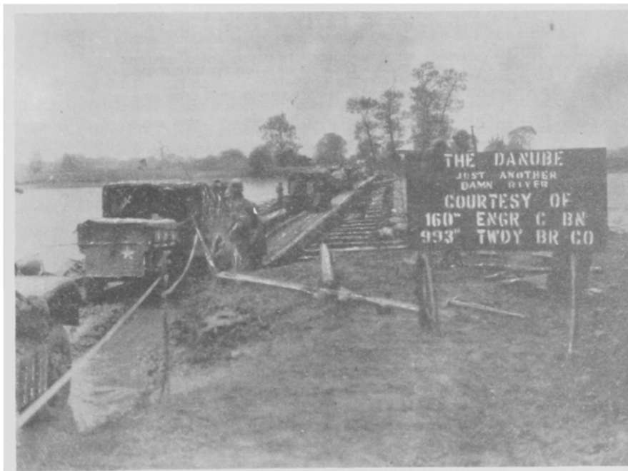
The treadway bridge over the Danube River
