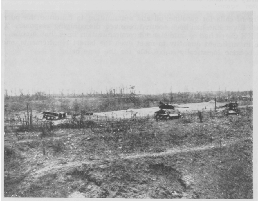
U. S. tanks at Fort Driant
