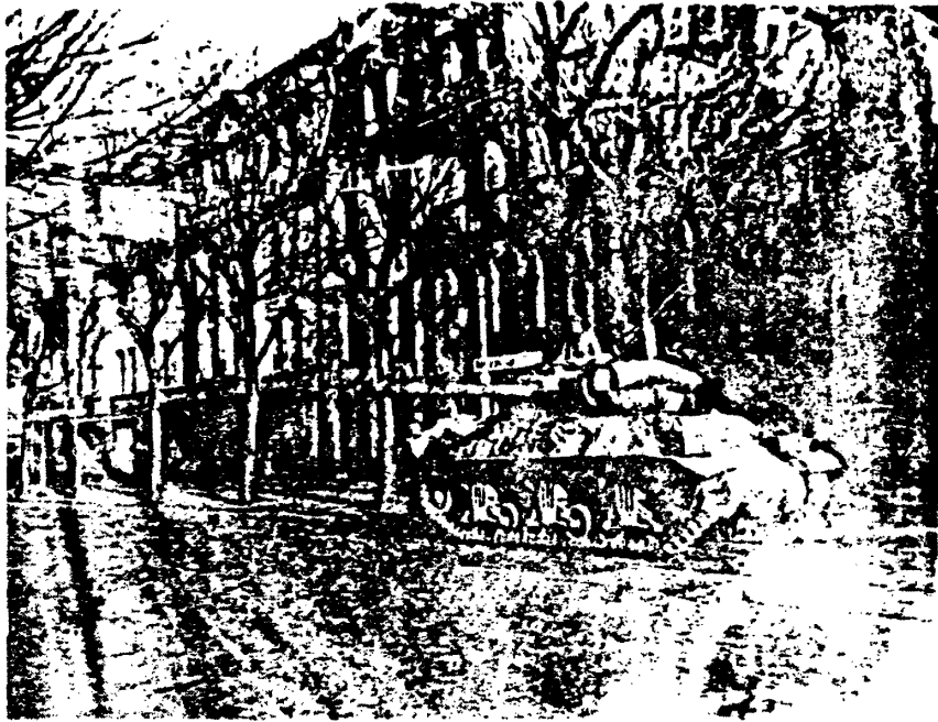
The First XX Corps Tank Destroyer to Enter METZ, 20 November 1944
