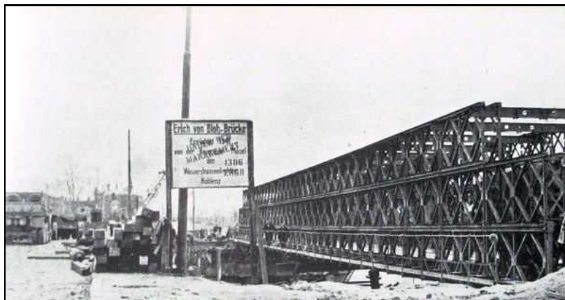
Double-triple Bailey provided permanent approach to and from Thionville.
