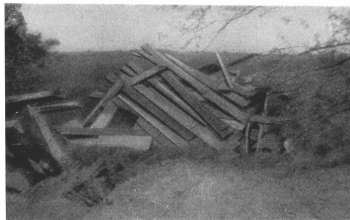
Bridge Failure under heavy Tank - Gouvey
